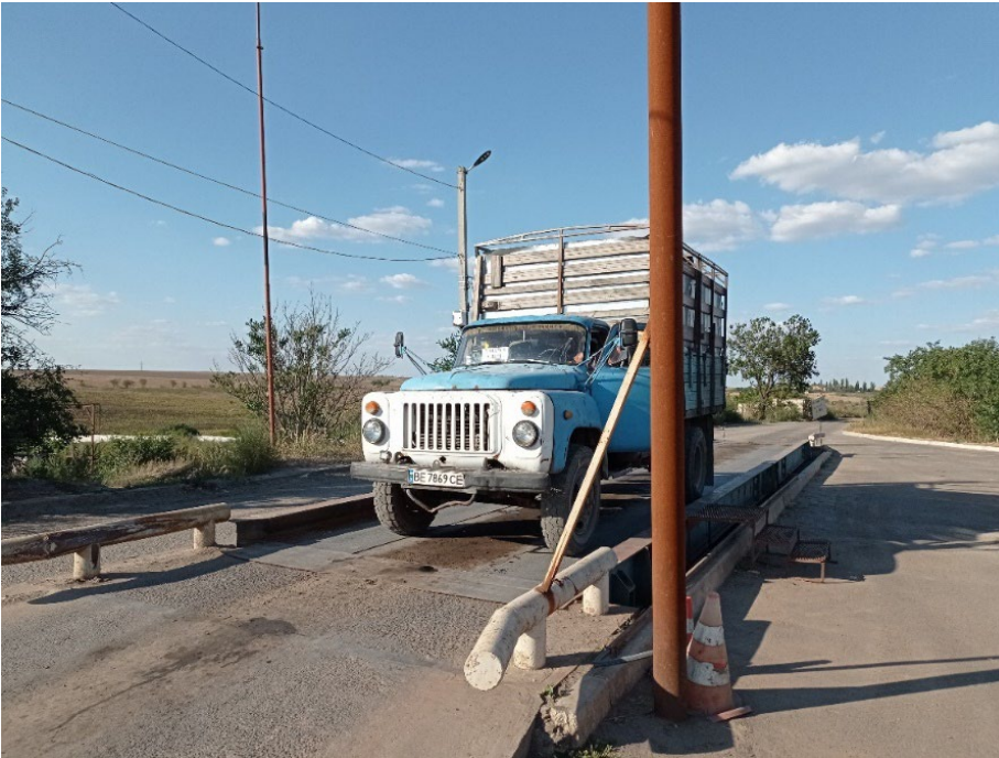
Figure 6-5 Weight bridge at the Mykolaiv landfill
