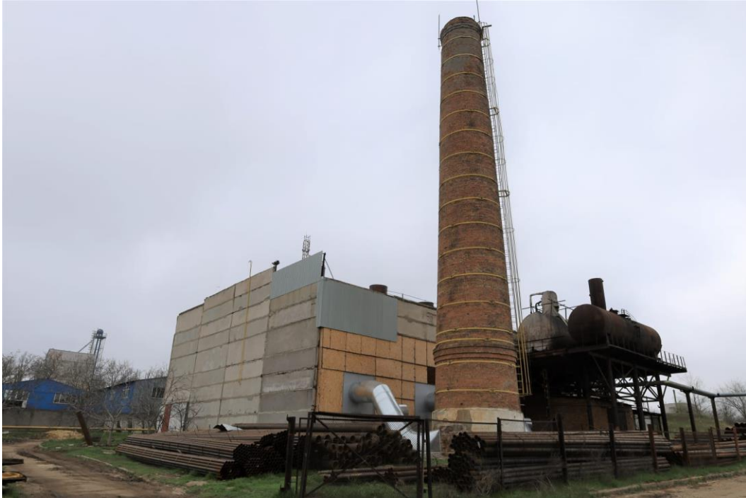
Figure 5-2 ... and the restored boiler house before the heating season.
